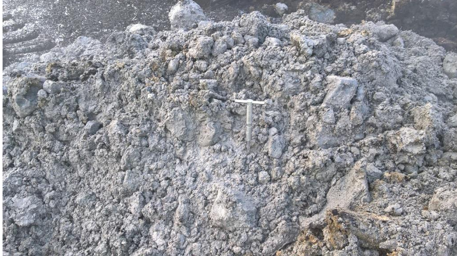
General view of the Very loose to loose silty SAND with numerous gravels and cobbles
